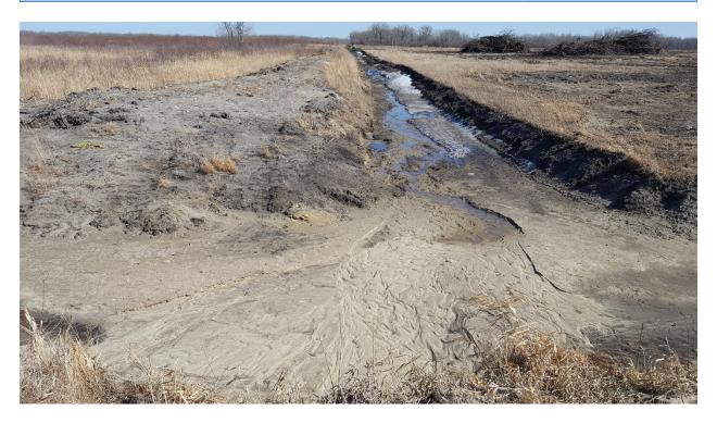
A large area of dramatic erosion problems was discovered along a ditch along 250<sup>th</sup> Ave SE, near the border of Red Lake and Polk Counties. Conversion of a large section of land from forest/pasture to cultivated land, along with a lack of a buffer, has caused severe erosion problems along the bank of the ditch and severe wind erosion.
